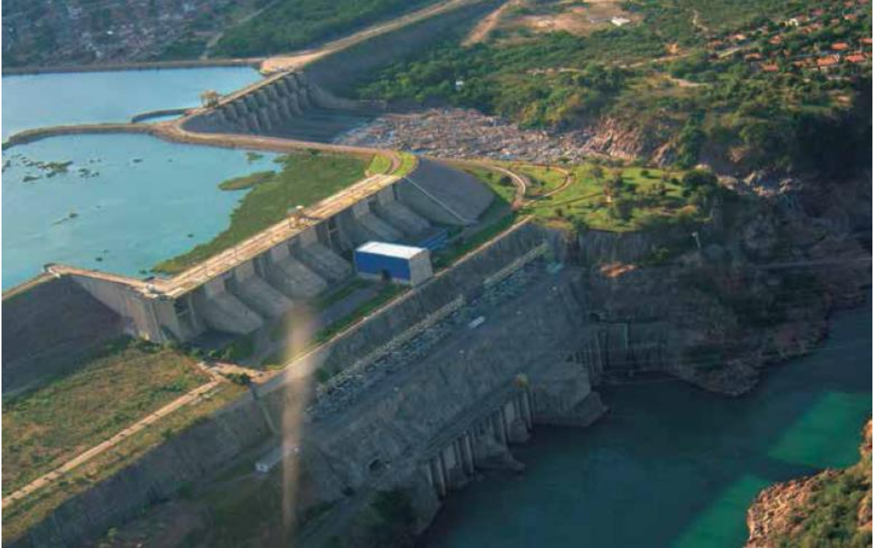
Hydroelectric dam in Brazil (Credit: Angela Linivo)
